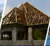
ROOF CONSTRUCTION & INSTALLATION
